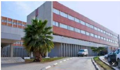
23 SEP 2024 LUBANGO CENTRAL HOSPITAL HOSTS I HOSPITAL CONGRESS
