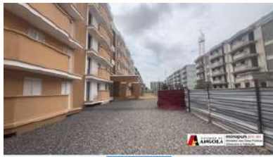
Lot 2 of the KK5600 project begins with the construction of 2,546 new homes.
