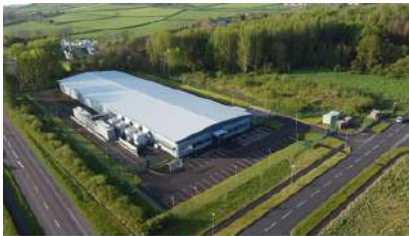
APRIL 28, 2026 Angola's National Government Data Center and Cloud will be inaugurated in Luanda.
